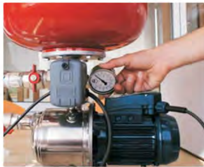
4) Remove the pressure gauge
