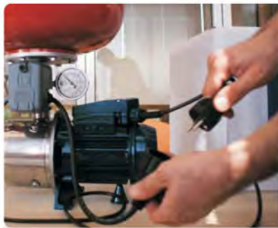
3) Disconnect the cable feeding the pressure switch
