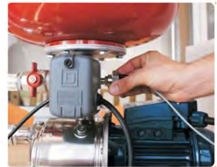
5) Install the pressure transducer
