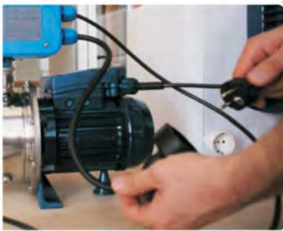
3) Disconnect the cable feeding the Pressure regulators
