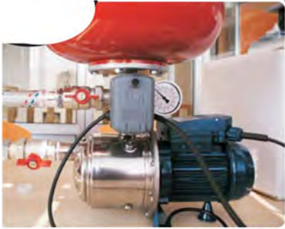
Old system controlled by pressure switch
