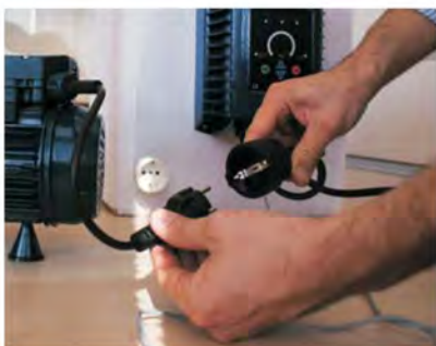
6) Connect the Inverter to the electric pump
