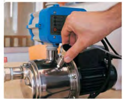
5) Install the pressure transducer
