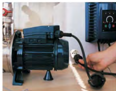
7) Connect the inverter to the mains
